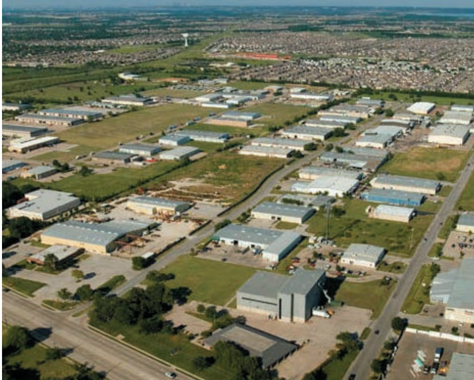
Oil States Industries sales, engineering & manufacturing facility | Arlington, Texas USA
